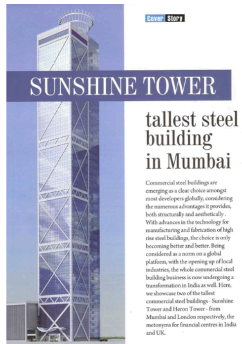
Figure 11: A page of magazine article on the tallest steel tower in India obtained from the Owner's website.
